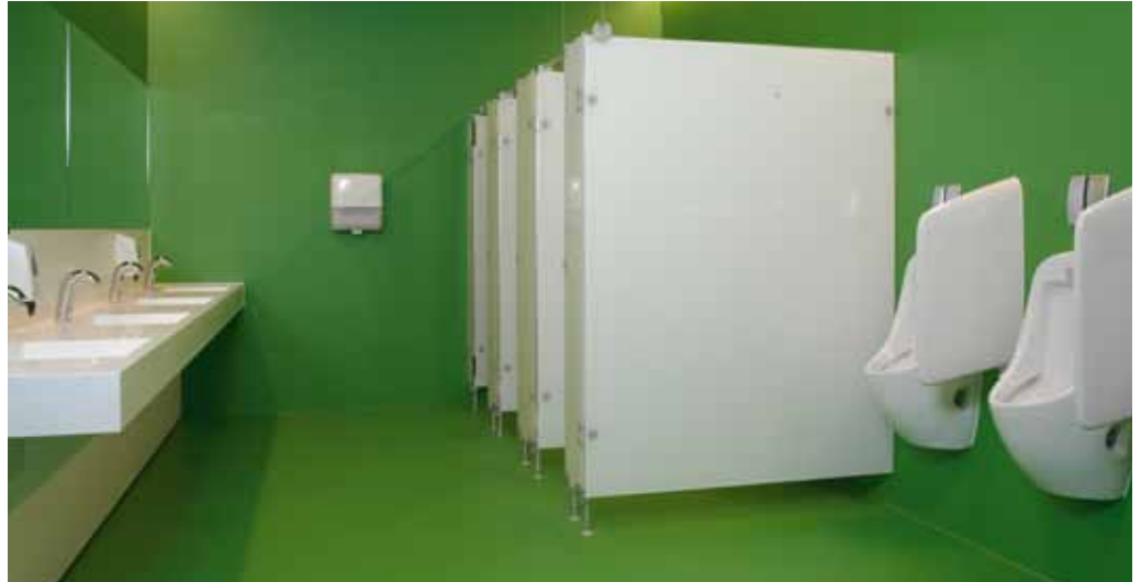
Our reference in Baar (Switzerland): zuwebe residential workshop facility
